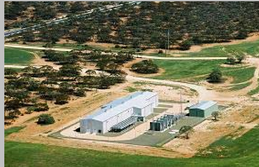
Berri Converter Station
