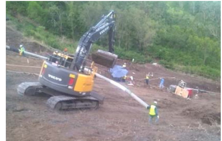
Repairing the Roma Brisbane Pipeline post floods
