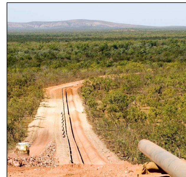
Pipeline stringing - Bonaparte Gas Pipeline
